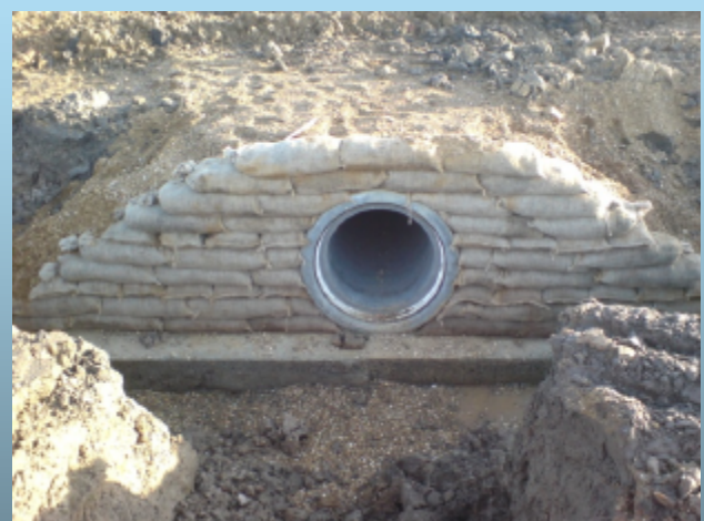
One of the Badger tunnels under construction.
