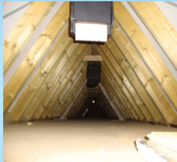
Bat loft within newly renovated barn
