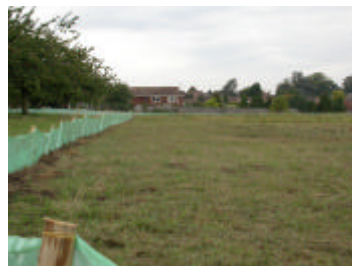
One section of the 3km of reptile proof fencing required at Fulston Manor Farm
