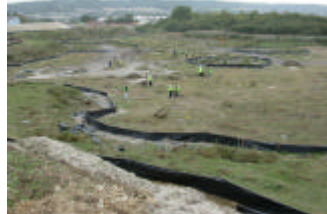
Holborough quarry showing ancillary workers and some of the extensive exclusion fencing
